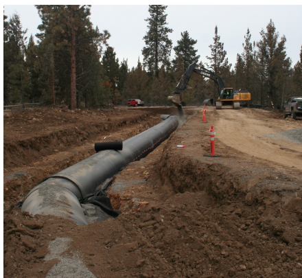
Laying pipe in Tumalo Irrigation District, February 2020. Photo credit FCA.
